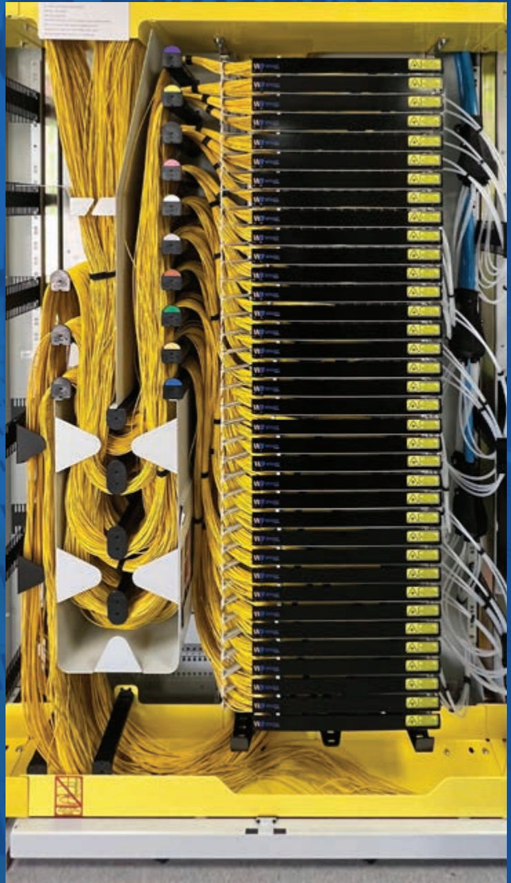
Example of bottom left cable entry and breakout for stranded fibre
